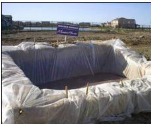
Plate 3-1 Typical concrete wash out areas
