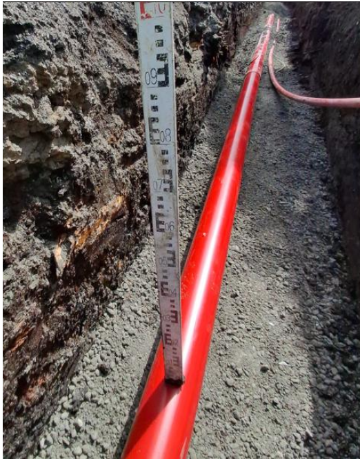
Plate 2-1 Typical Single Cable Trench View
